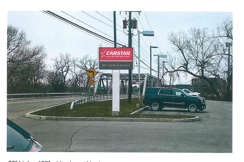
60" high x 100" wide sign cabinet radius endcap set on 8" x 8" square steel pole (48" into the ground and 12 feet out of the ground) Flat poly faces with vinyl graphics 40 sq feet allowed from the Town Sign is at 40 sq feet From the ground to top of sign is 17 feet
